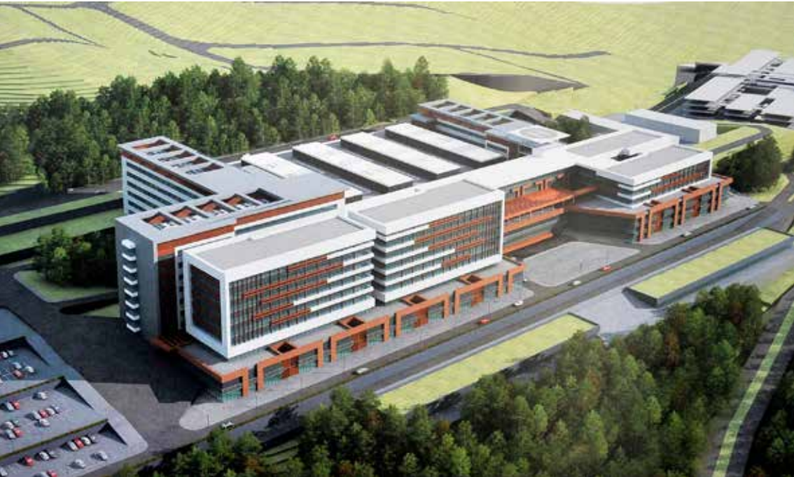
KOCAELİ CITY HOSPITAL
