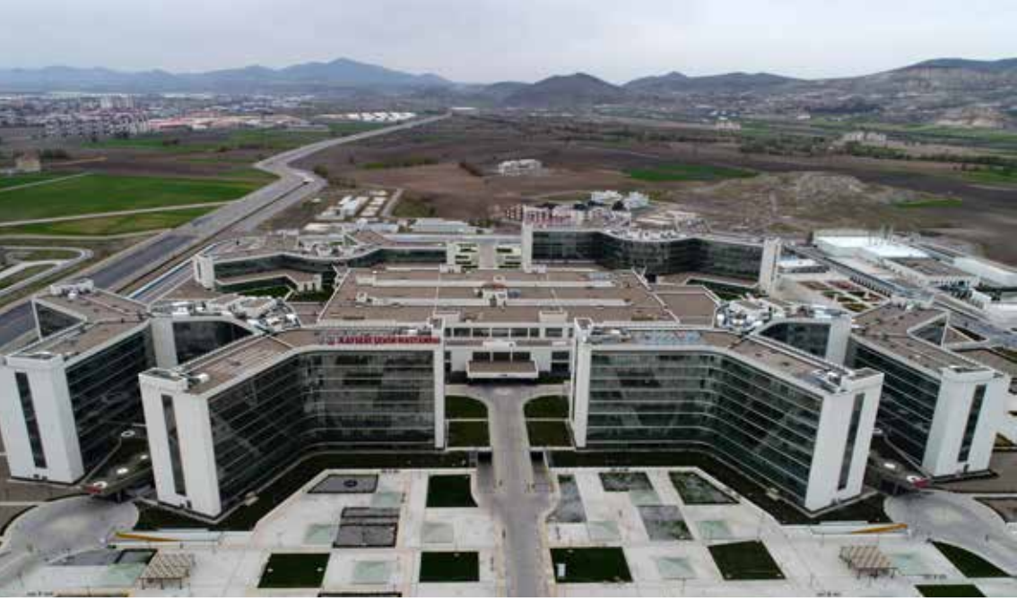
KAYSERİ CITY HOSPITAL
