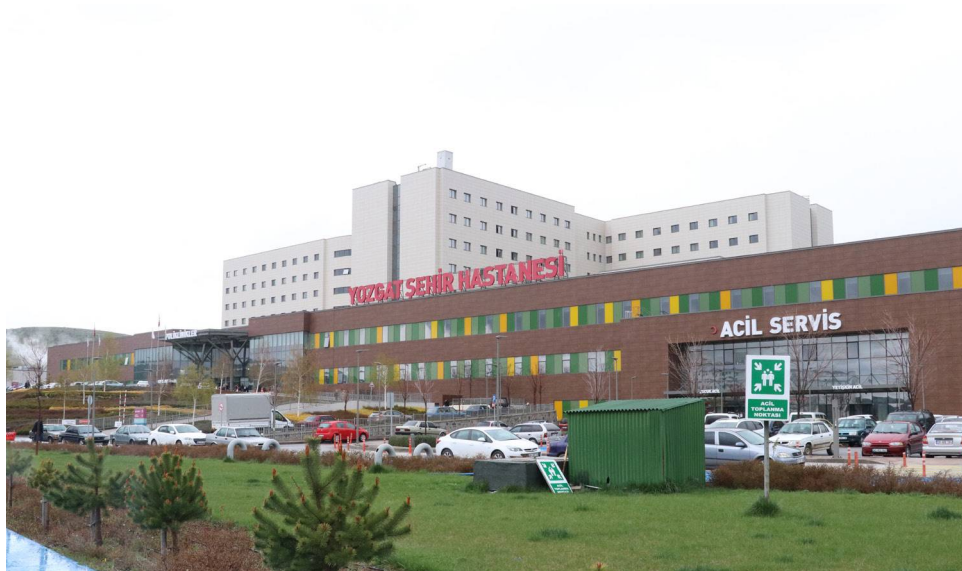
YOZGAT CITY HOSPITAL
