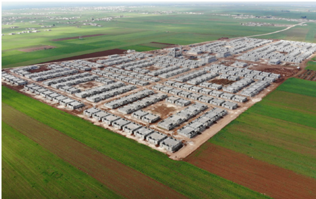
An example of the briquette house sites currently under construction at various locations in northern Syria (May 20, 2023).
