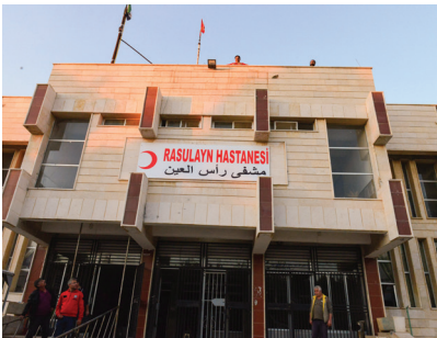
Ras al-Ayn Hospital
