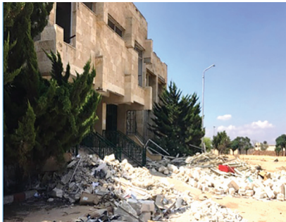
Azaz Vatan Hospital Before the Renovation
