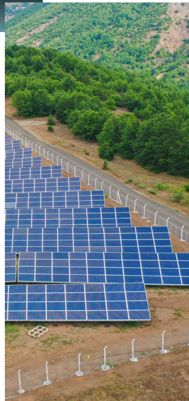
Solar power plant, Akkus/Ordu
