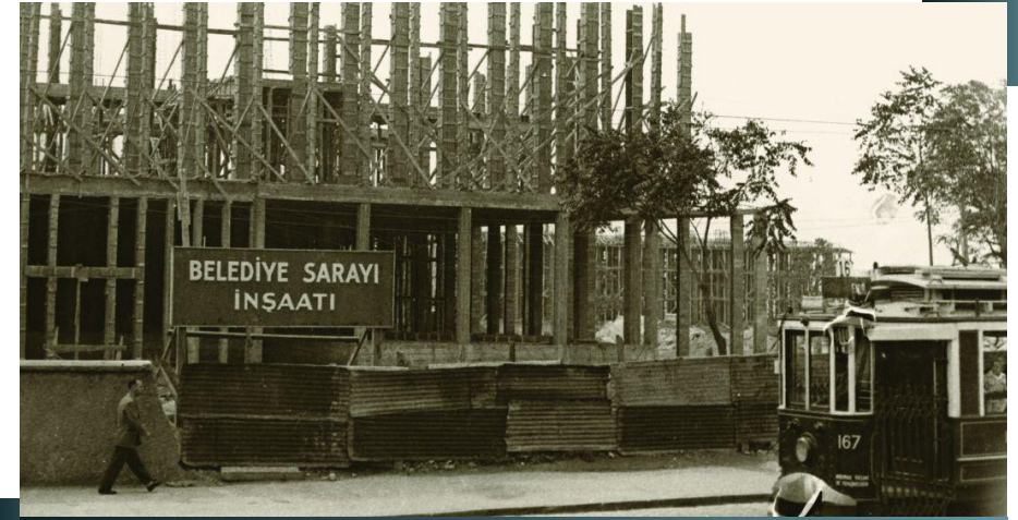
Construction of Istanbul City Hall and the tram passing in front of it, Istanbul
