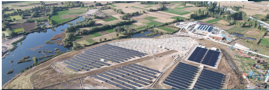
Solar Power Plant Project, Sakarya
