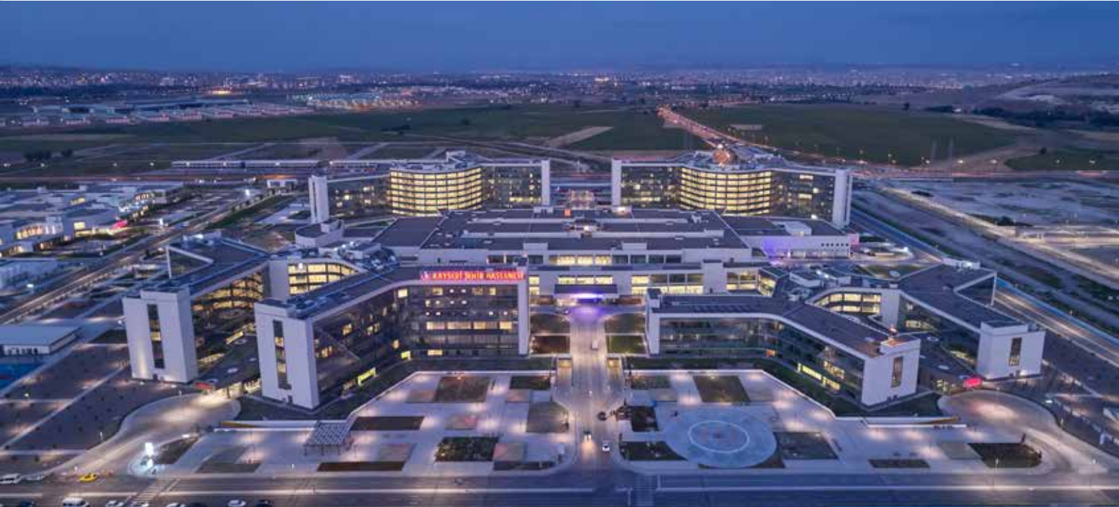
KAYSERİ CITY HOSPITAL
