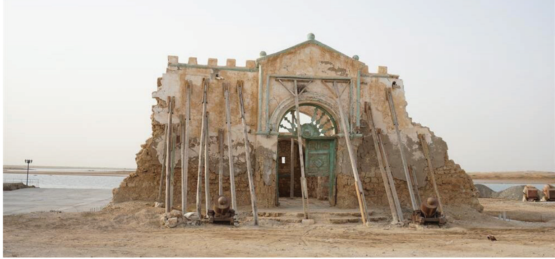
Preservation Building Restoration on-going
